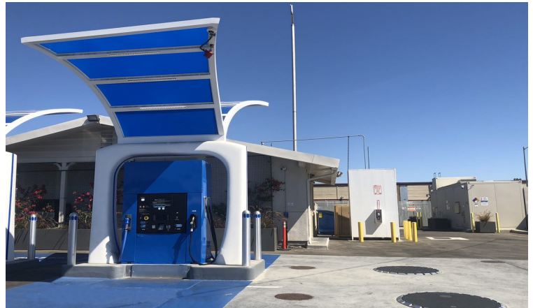
Hydrogen Fueling Station - Vacuum Insulated Lines
