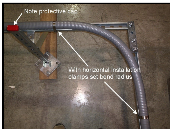
Figure 12 - Techniguard B-Series VJP installation showing proper clamp placement.
