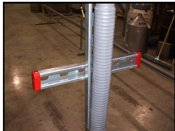
Figure 4 - Structural channel used for mounting vertical routing.
